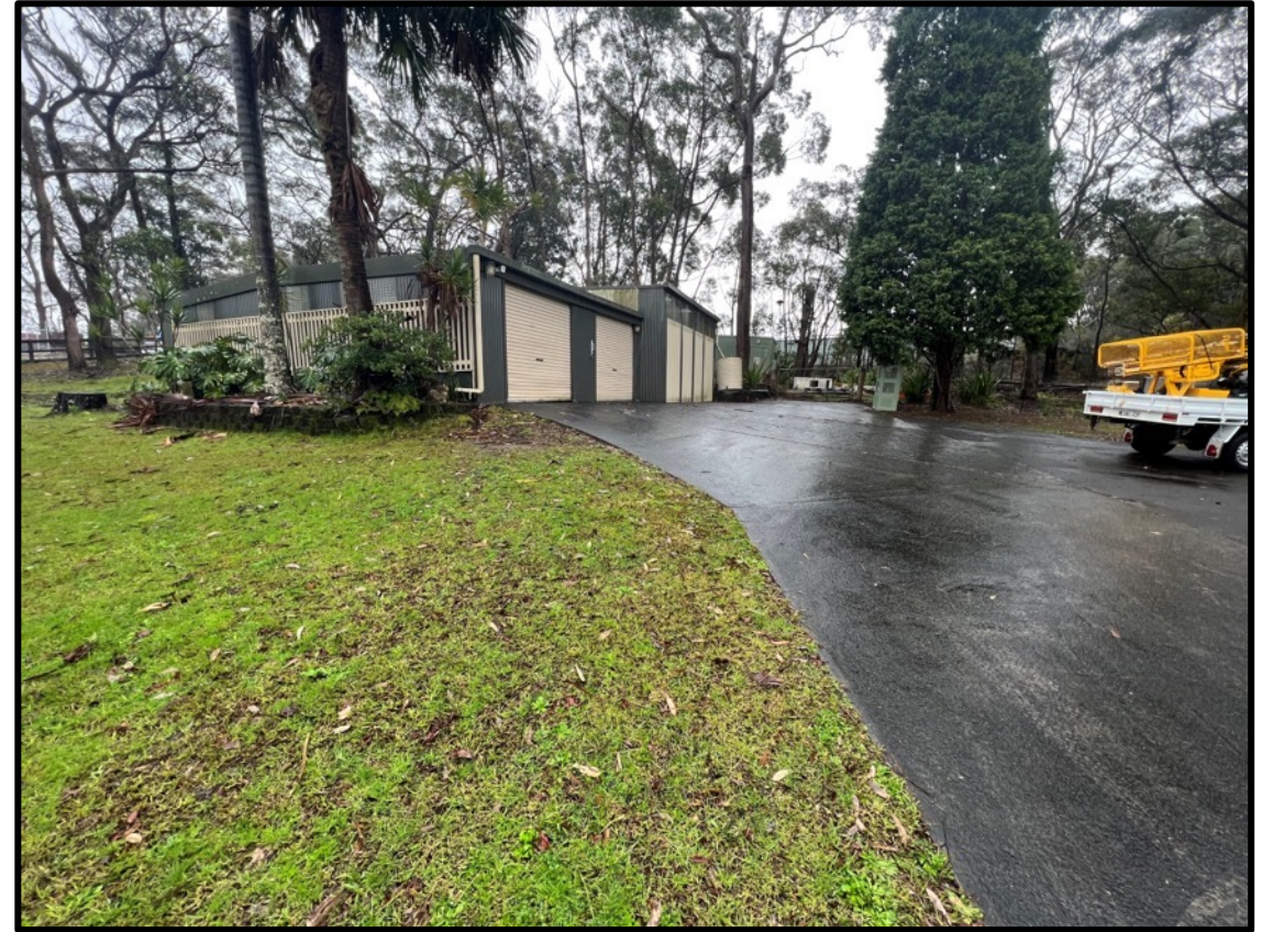
Figure 9. Metal sheds within the northwestern portion of the site.
